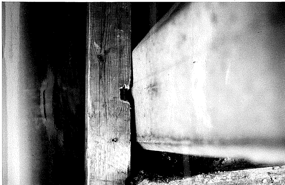
Fig. 3.15 Notch cut in bracing to allow piano wire to pass by
