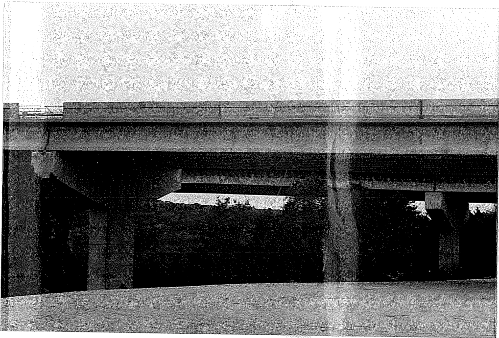
Fig. 3.11 Traffic rail above beam H-01
